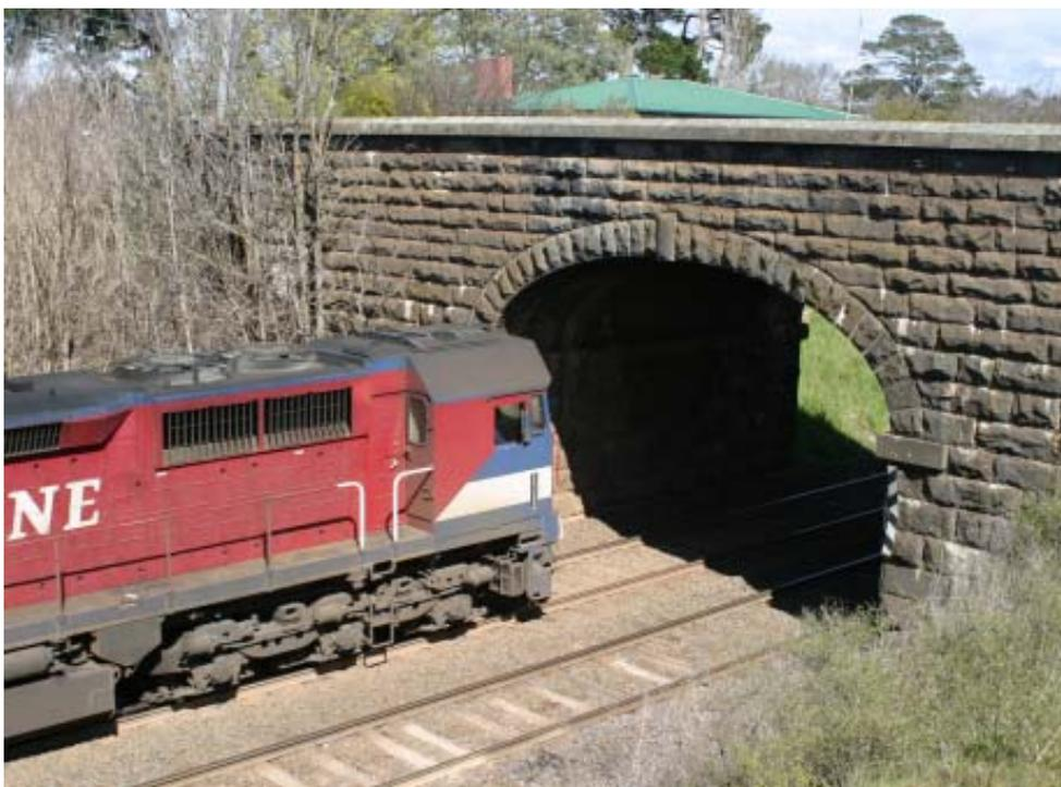
Narrow clearances under arched bluestone overbridges are another reason offered by DoI for singling long sections of the Bendigo line. Here, N473 seems to have little trouble clearing the Dalysesford-Malmsbury Road overbridge at the line speed of 130km/h with a passenger service on Tuesday 7 October 2003. Bob Wilson
