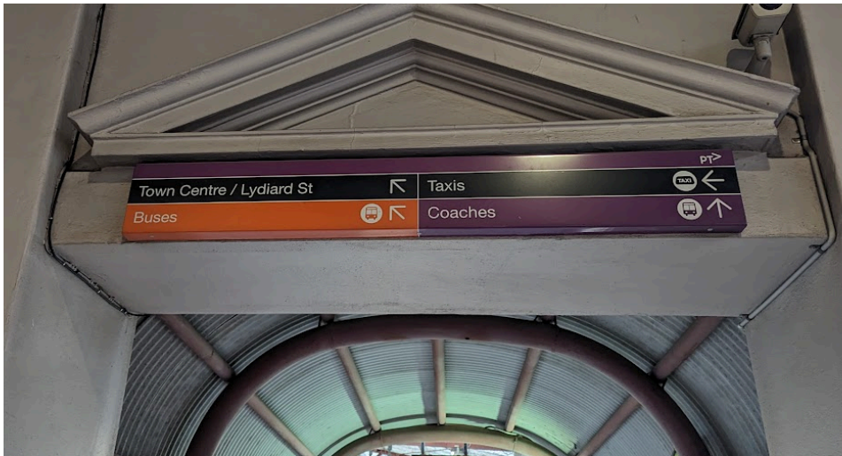
An example of incorrect wayfinding at the coach bay exit of platform 1. It points users in the wrong direction for buses and does not indicate pram/wheelchair access to platform 2
