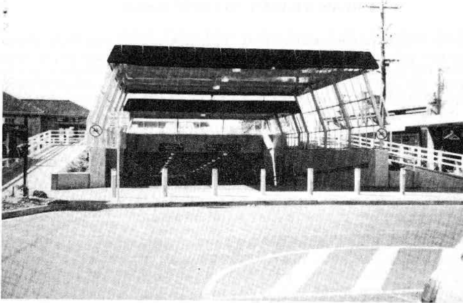
Top: An impressive entrance to the rebuilt Werribee Station is adjacent to the shopping centre. As well as ticket facilities, several modern shops nestle in the spacious subway.
